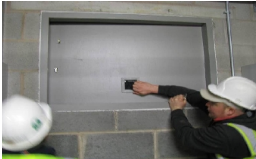
High Level Access Door to Silo
