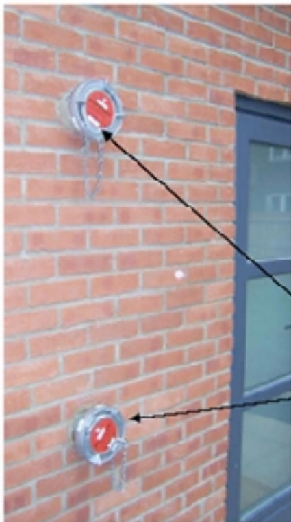
Pellet Fill and Exhaust Pipes (Storz A fitting) on outside of Pellet Silo
